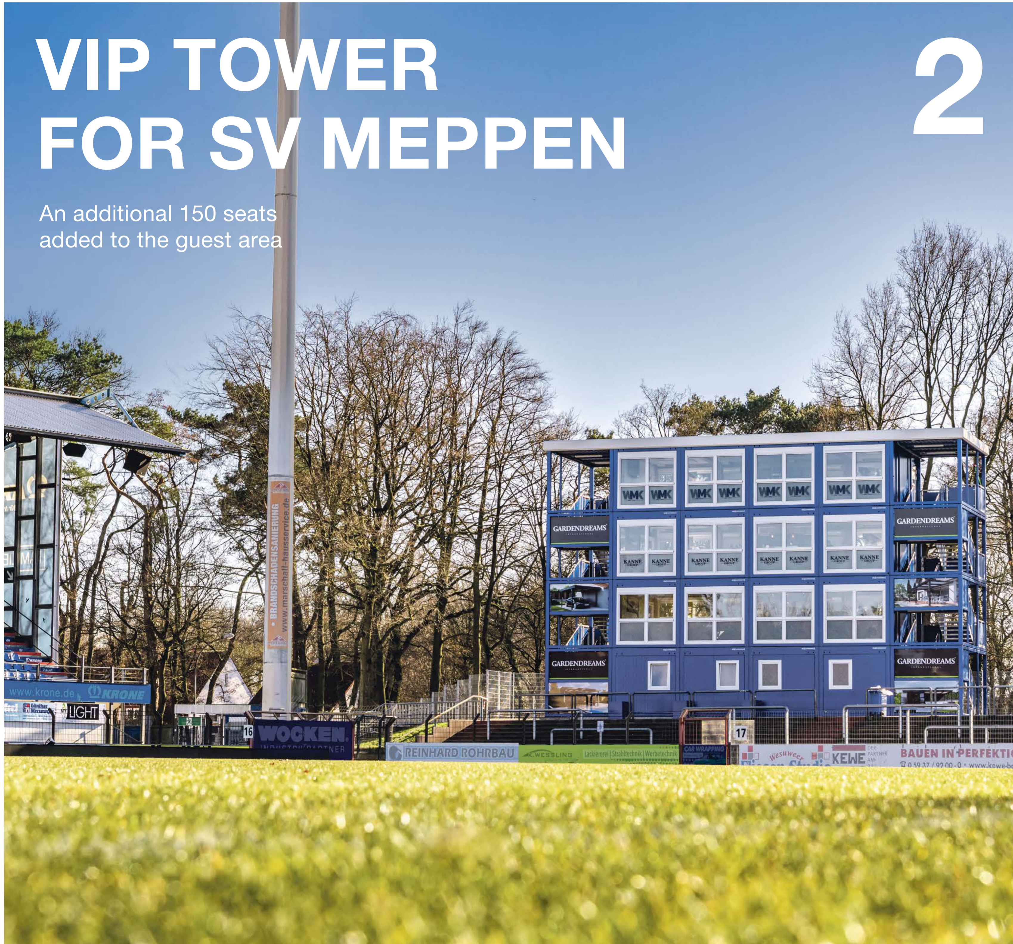
The four-storey system offers 432 m 2 of space for guests and function rooms.
