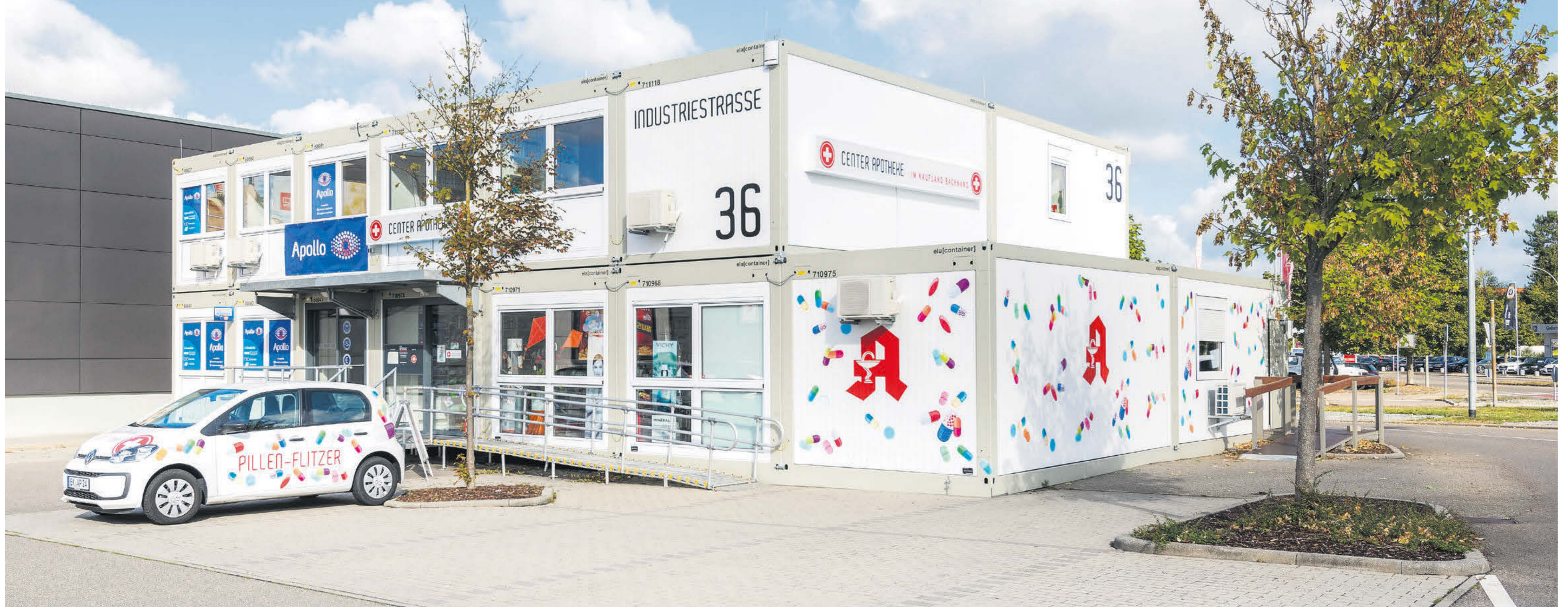
The shopping centre is undergoing renovation, but the opticians and pharmacy carry on their business in ELA retail spaces.
